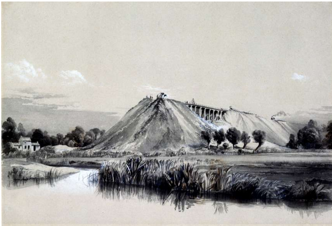
Figure 2 End tipping of material during the construction of the 15m high Wolverton embankment on the London to Birmingham Railway circa 1835. Note the tipping truck on the top of the embankment.
