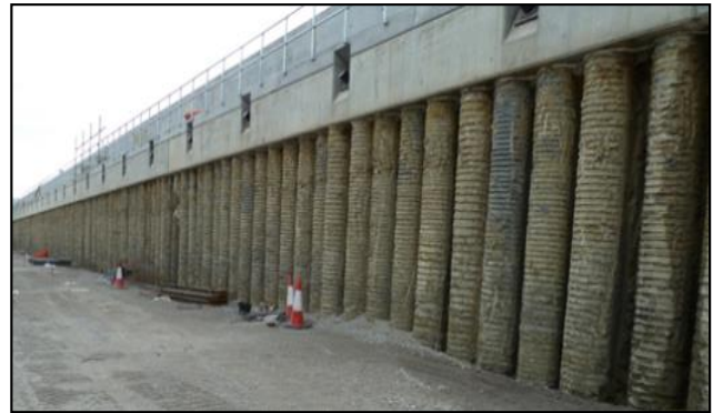
Figure 2 Retaining wall prior to being faced
